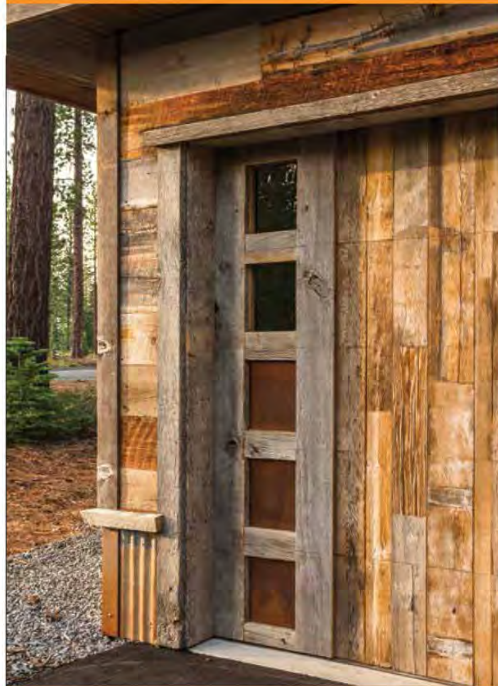
THIS PAGE: Steel details accent the garage. OPPOSITE PAGE, FROM TOP: An outdoor dining area is adjacent to a board-formed concrete-surrounded fireplace for chilly nights | Parts of two barns were used for the exterior wood.
